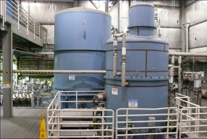
4600W @ 2.1K Refrigerator & 1st set of Cold Compressor (2K Cold Box), 245 g/s
