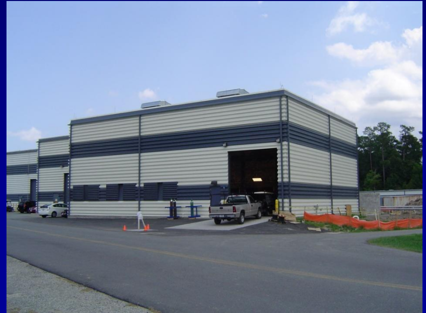
CHL #2 Building (March 10)
